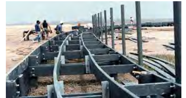
High density polyethylene bridges replacing treated timber
