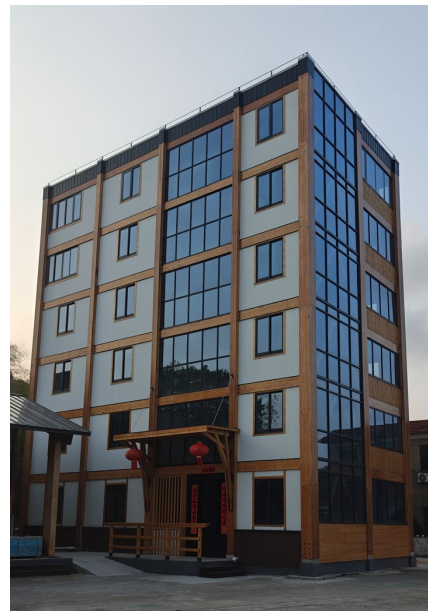
Fig.3. World's first seven story engineered bamboo tall building – the Ninghai Bamboo Tower
