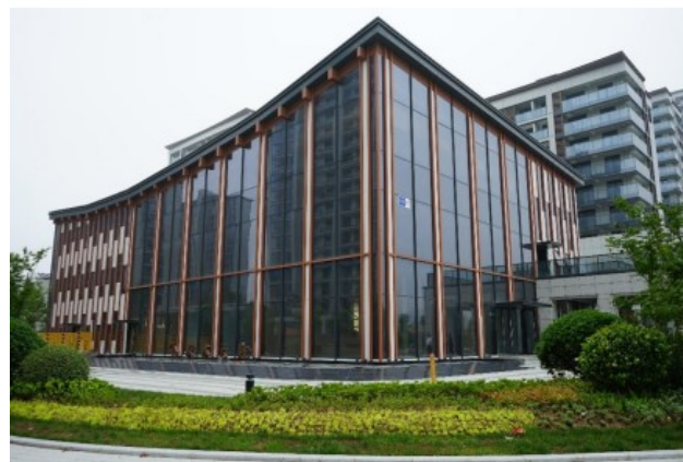
Engineered bamboo building — Ninghai Double Water Low Carbon Community Center
