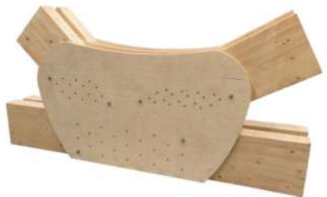
Plywood as connection plates on a timber truss joint
