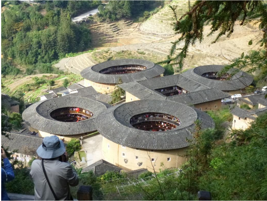
Traditional Tulou buildings with mud brick exterior over timber frame.
