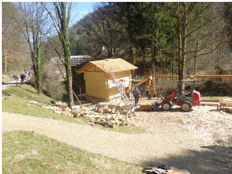
Construction of historic wooden mill.
